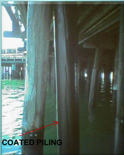
STEARNS WHARF, SANTA BARBARA ACZA TREATED TIMBER PILE
