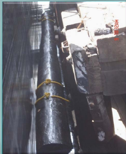
PORT OF LOS ANGELES, PRESSURE TREATED TIMBER CAMEL LOG
